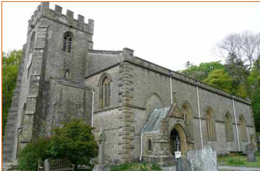
Clapham Bridge ( figure 28 ), grade II listed –
