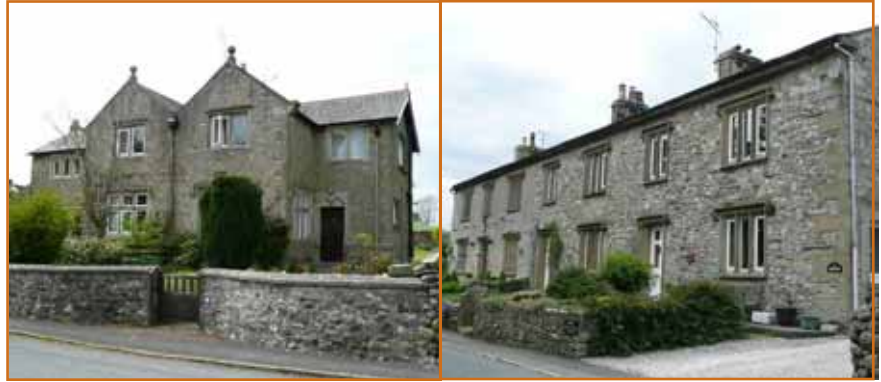
Figure 52: Buildings on Station Road (photos © Gaby Rose, YDNPA, 2010)
