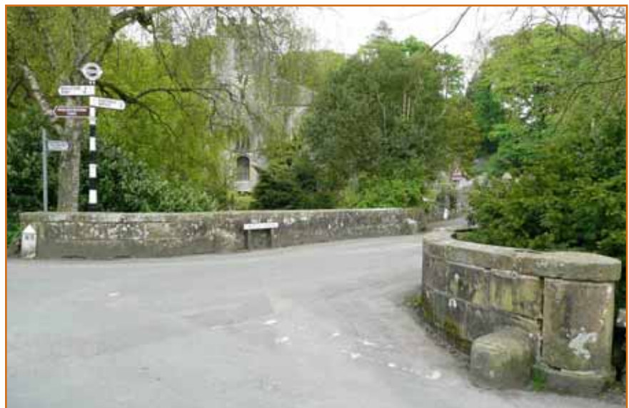
Church of St. James ( figure 27 ), grade II listed –
