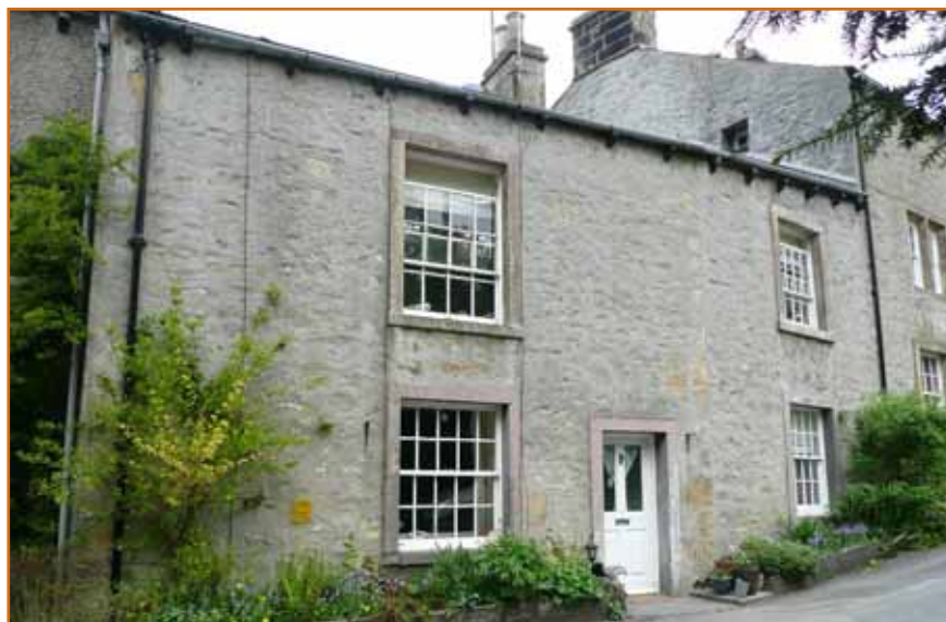
The Beeches (upper cottage) ( figure 38 ), grade II listed –
